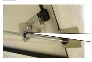
Check that the doors close easily and that the locks are correctly adjusted. If necessary, the height of the glide angle can be adjusted
